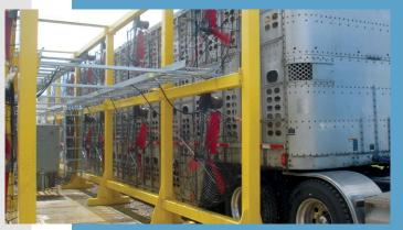
Combined water sprinkling and ventilation system. Source: Sherbrooke Research and Development Centre, AAFC
